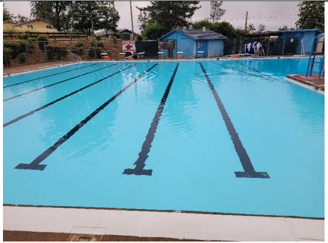
Figure 7. Paradise Pool newly refilled after resurfacing
