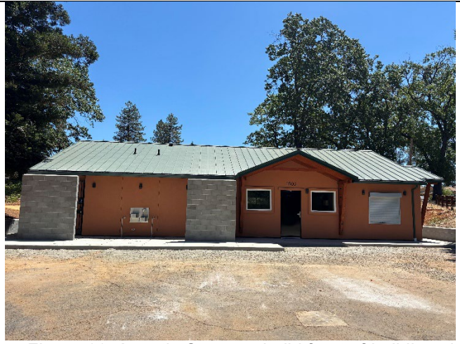
Figure 11. Aquatic Center rebuild front of building view
