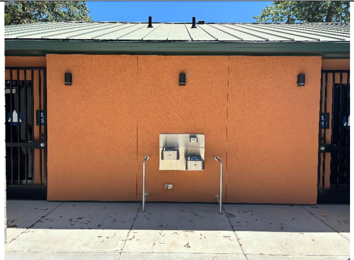
Figure 13. Closeup of restrooms and drinking fountain
