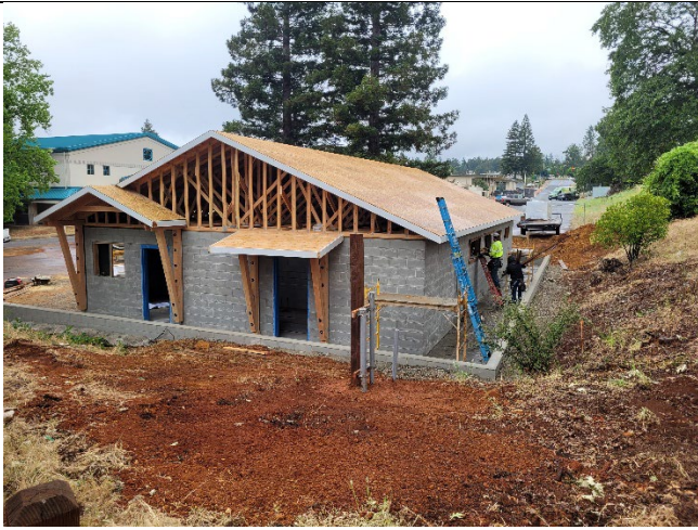
Figure 10. Aquatic Center being rebuilt in May 2026
