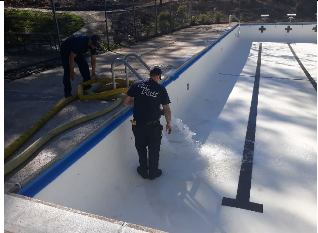
Figure 3. CalFire refilling the pool after Camp Fire cleanup
