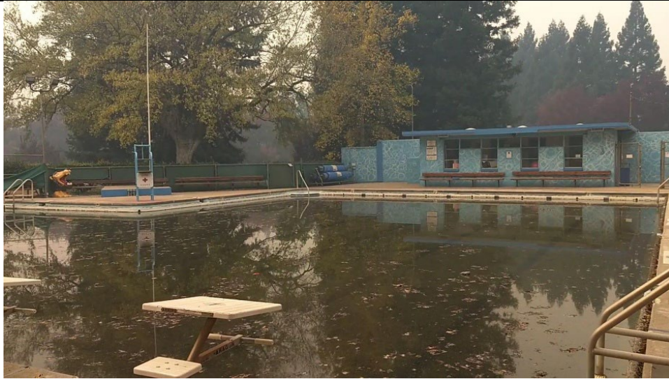
Figure 1. Paradise Pool post Camp Fire
