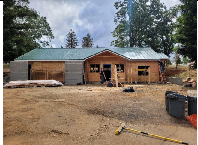
Figure 9. Aquatic Center being rebuilt in May 2026
