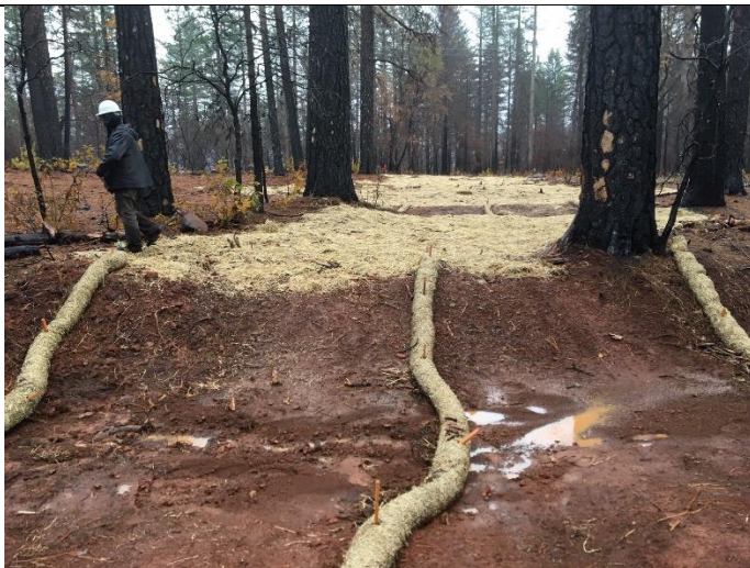
Figure 1. PG&E completed work at Coutolenc Park in December.
