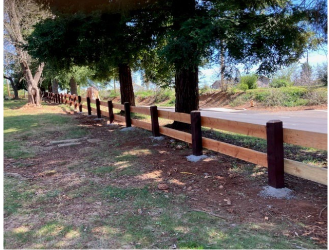
Figure 2. The Aquatic Park fence after the maintenance crew fixed it.
