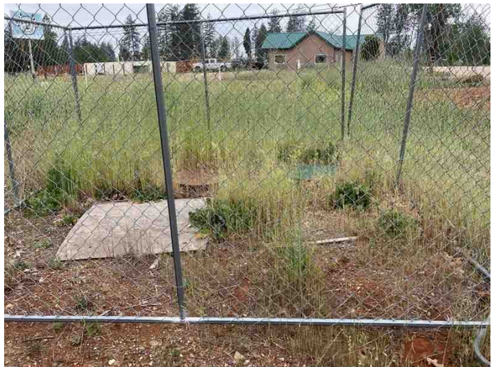
SEPTIC TANK LIDS - EXTRAORDINARY ASSUMPTION MADE THAT TANKS ARE NOT OPERATIONAL
