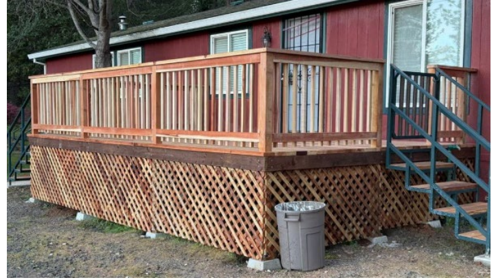
Figure 2. The deck at the Paradise Lake House after repair.
