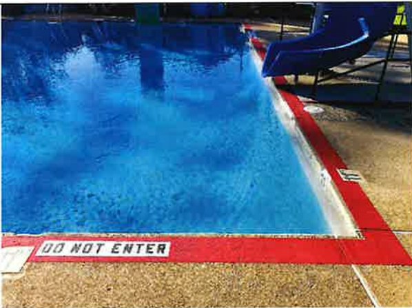
Figure 3. The pool deck boards after they were repainted for the upcoming swim season.
