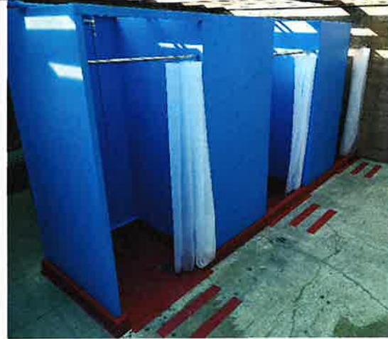
Figure 2. Maintenance removed the rust and repainted the women's showers at the pool, and they are looking great.
