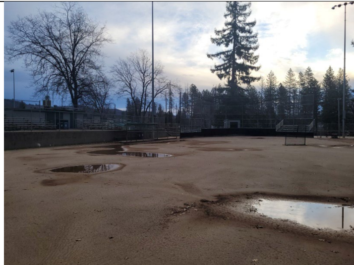
Figure 8. Heavy rains at the Ball Park have delayed baseball season.
