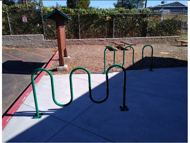
Figure 10. The Maintenance crew added bike racks at the TARC.
