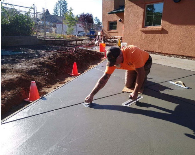
Figure 9. Park Supervisor Cobb laying new cement.
