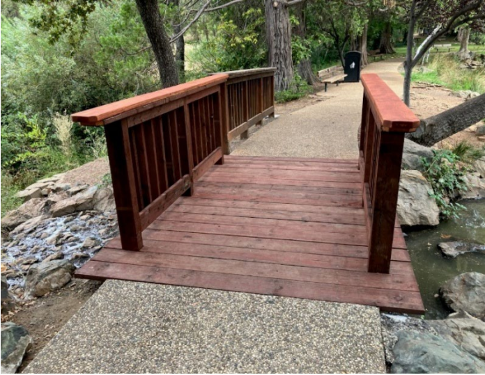
Figure 1. The new bridge at Aquatic Park.
