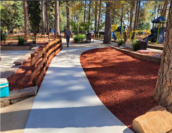
Figure 3. The sidewalk at Bille after repaving.
