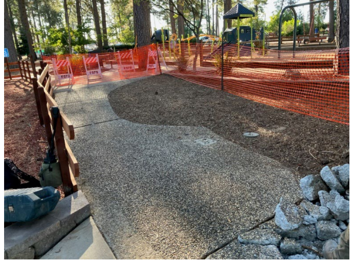
Figure 2. The sidewalk at Bille before repaving.
