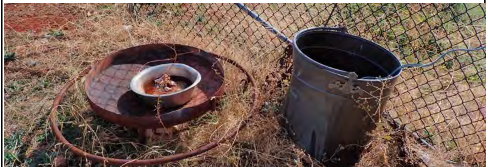
Image 21. View of rusted materials within the fenced in area.
