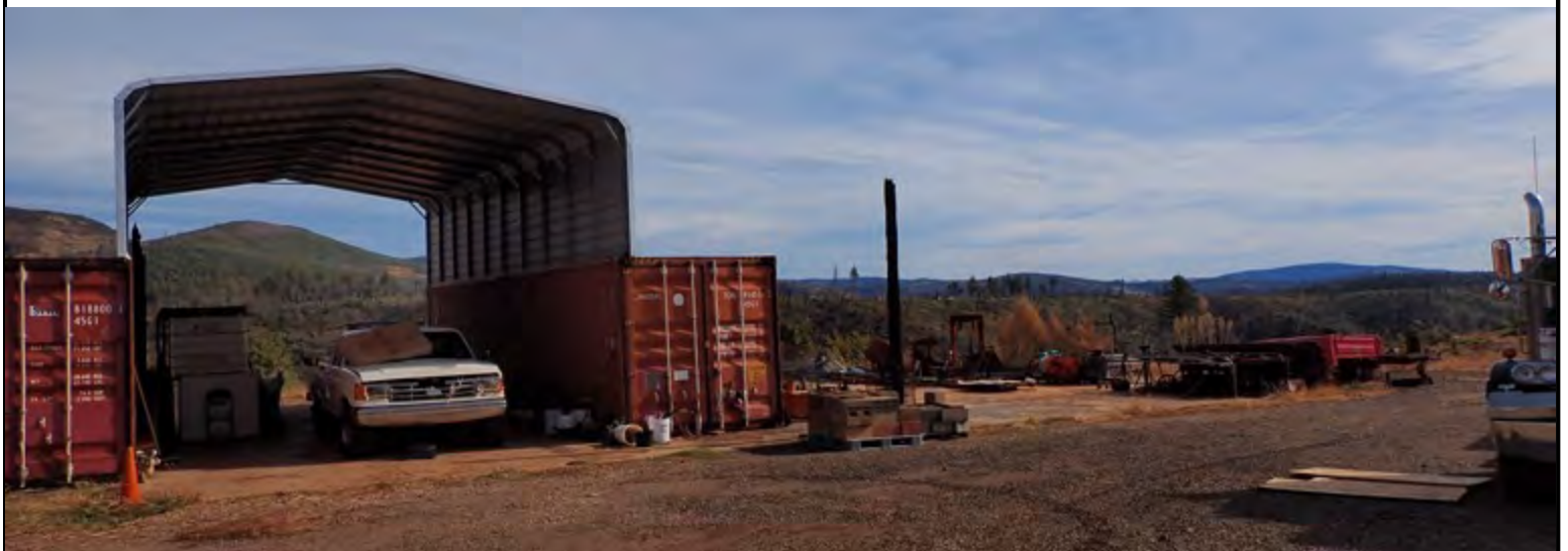
Image 47. Carport observed on paved slab, appeared to be used as a shop, with view of shipping units and additional equipment.
