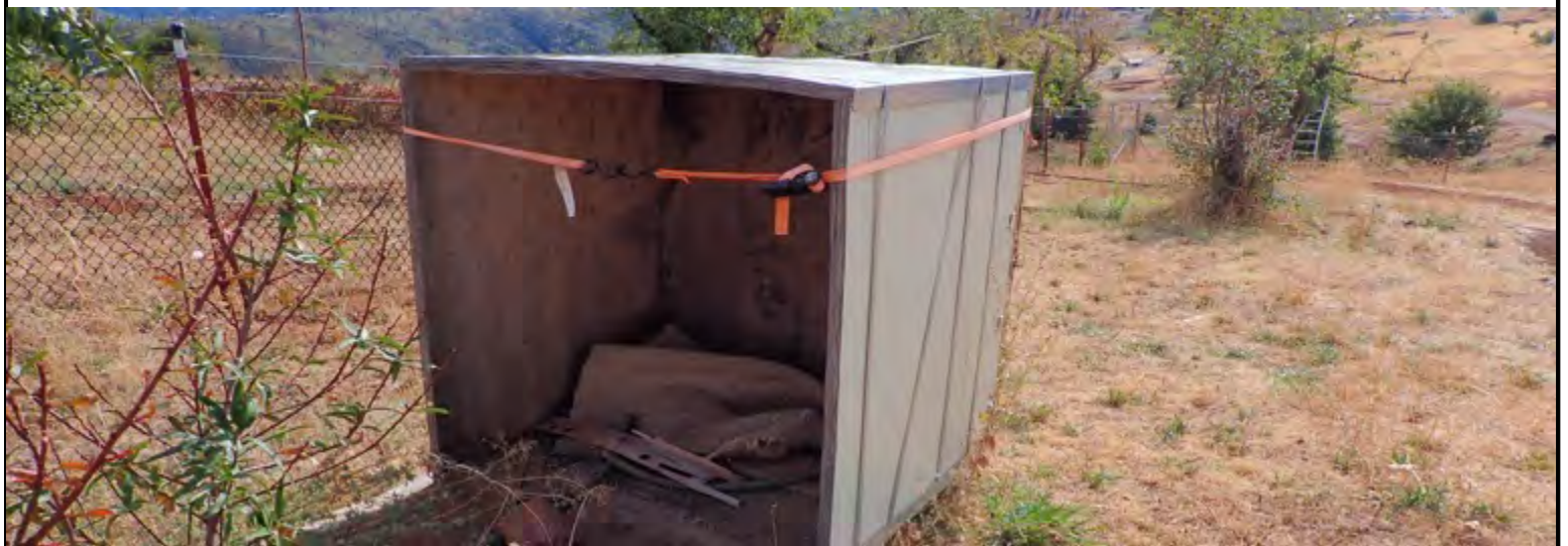
Image 20. Structure within fenced in area for canine shelter.
