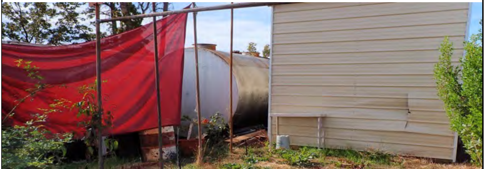
Image 8. Elevated tank as well as additional equipment and materials near the metal shed.
