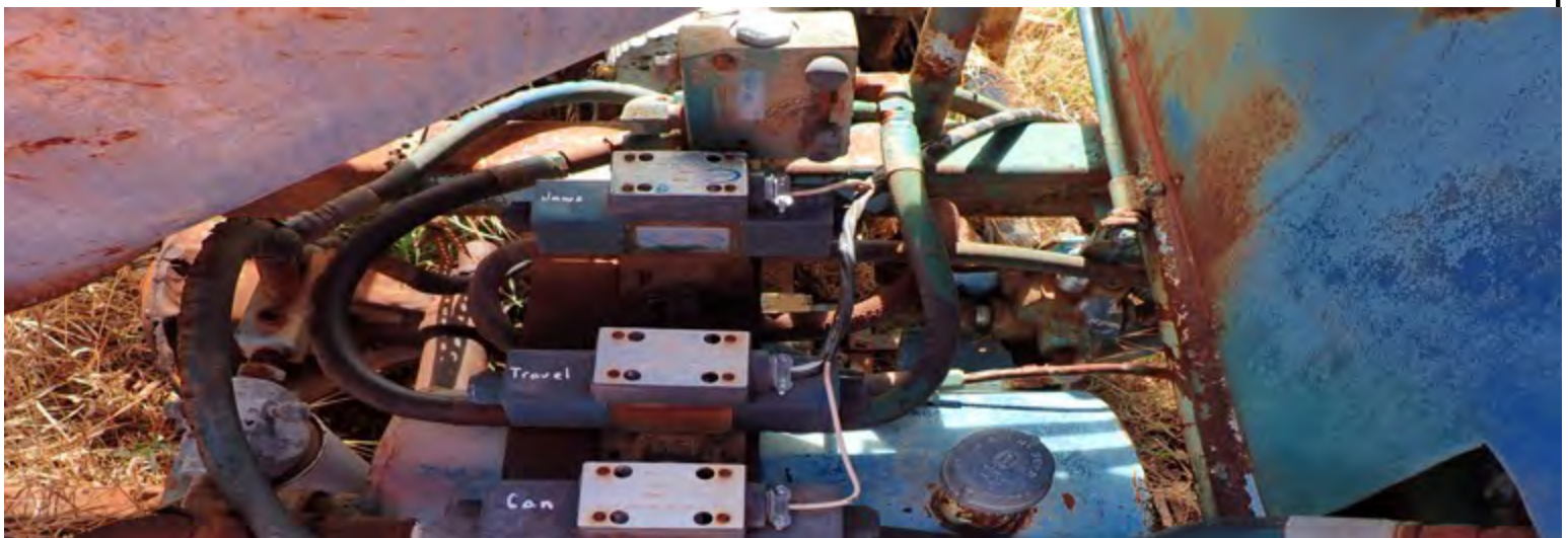
Image 27. Rusty piece of equipment located on the subject property.
