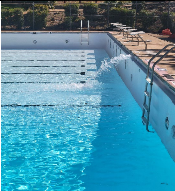
Figure 14. The resurfaced pool being filled.
