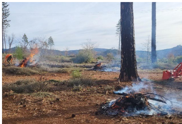
Figure 2. Maintenance Crews burning debris at Noble.
