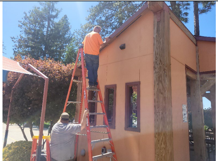
Figure 4. The Maintenance Crew is starting to repaint and stain the TARC. The BBQ area before.
