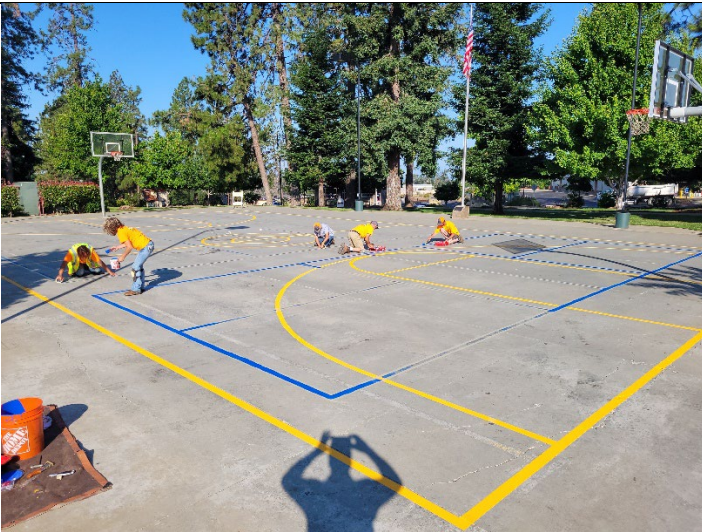
Figure 7. During the paint job.
