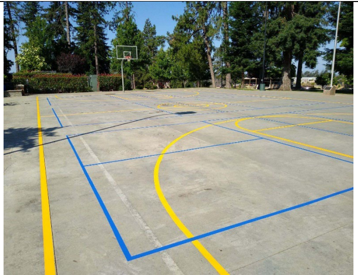
Figure 8. After the completion on the paint job.
