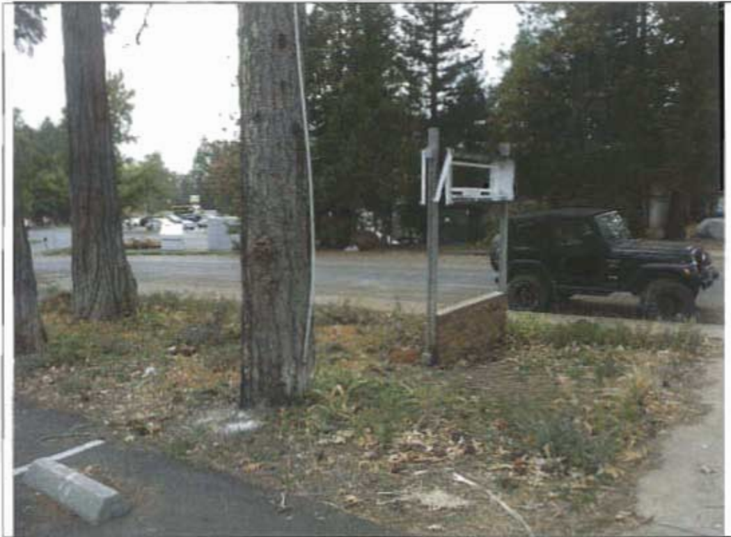
View SW toward Lakeridge Circle showing curb gutter and sidewalk. (296)
