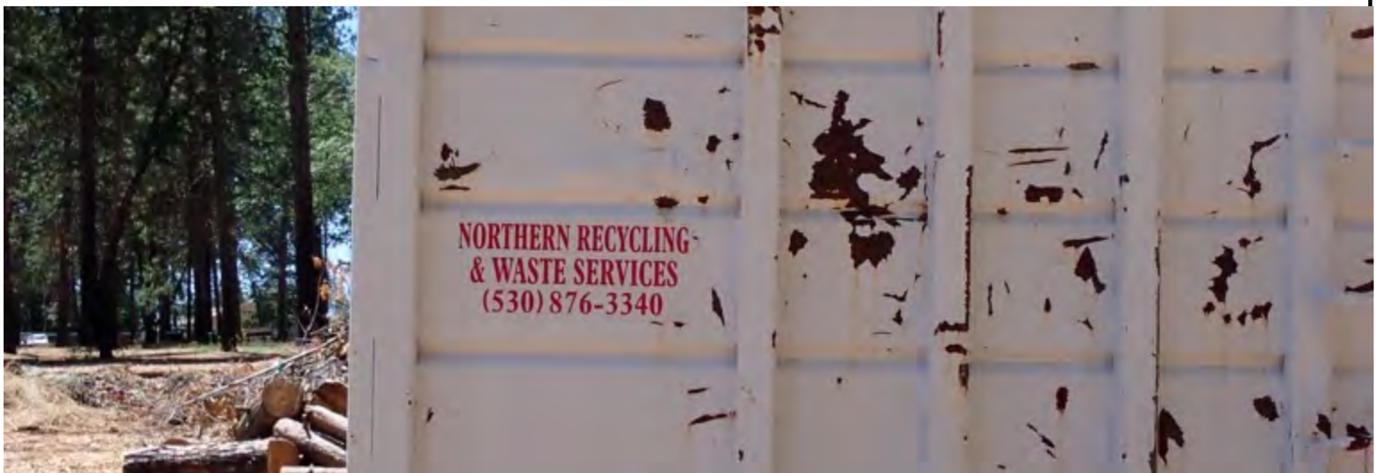
Image 33. Dumpster and cut trees stored onsite.
