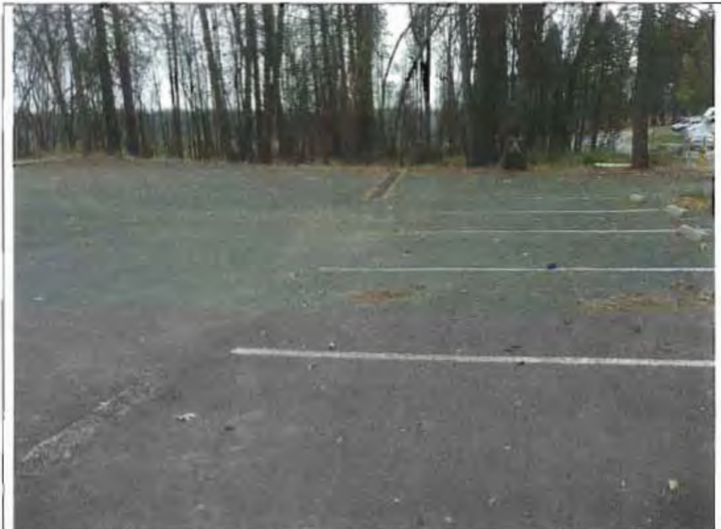
Looking south from western portion of lot showing parking lot and drainage. (297)
