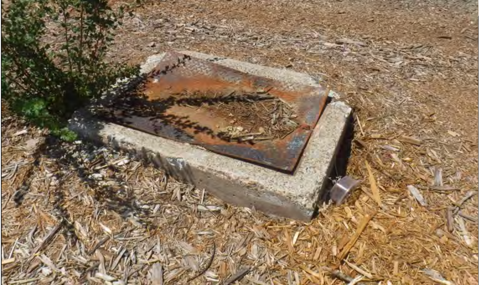
SITE PHOTOGRAPHS – JUNE 7, 2021 LAKERIDGE PARK PROJECT EAST OF LAKERIDGE CIRCLE AND WEST OF DOGTOWN RD, MAGALIA, CA
