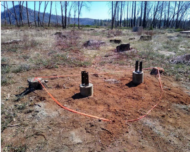
Figure 6. Footings for sign at Lakeridge Park.
