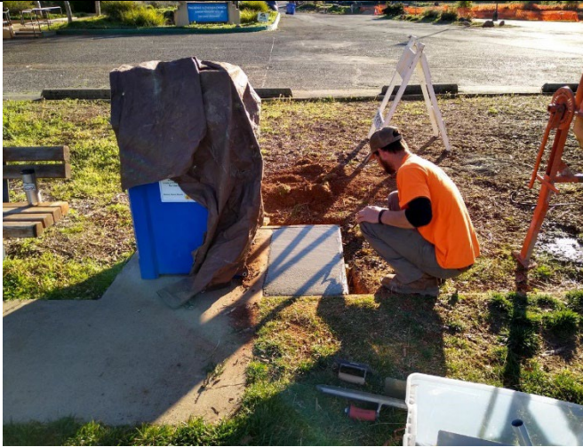
Figure 4. New Trash/Recycle Bin at TARC.
