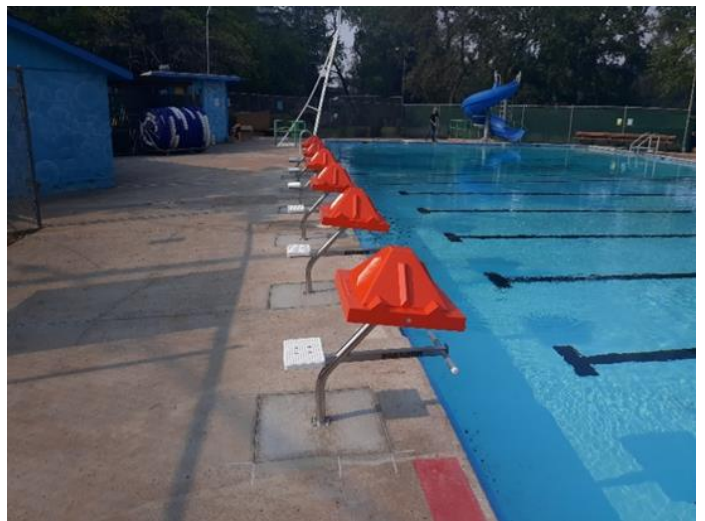
Figure 4. Newly installed Pool Starting Blocks.
