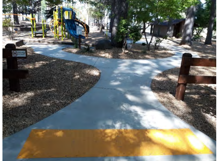
Figure 2. Sidewalk improvements at Bille Park
