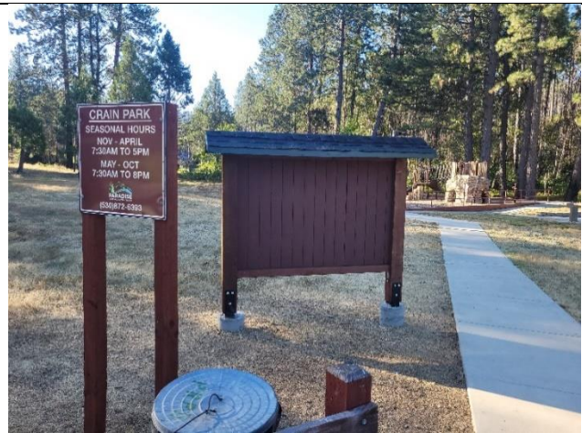
Figure 16. Completed welcome sign kiosk at Crain Memorial Park.
