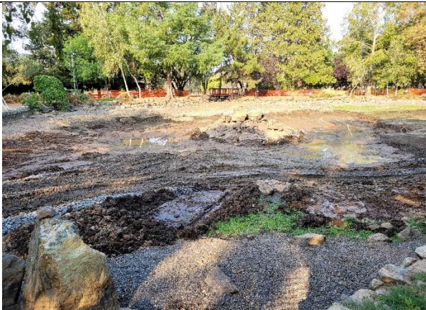
Figure 3. The Aquatic pond after the cleaning was done.
