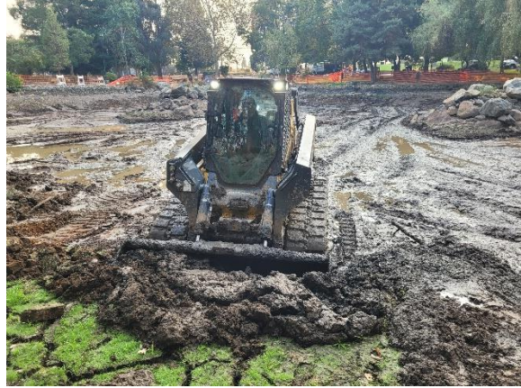
Figure 2. Ray scraping up sludge on the floor of the pond.
