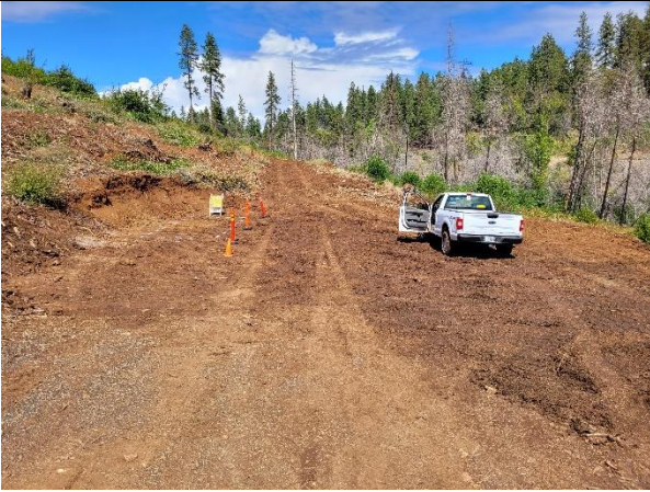
Figure 19. Oak Creek after debris removal
