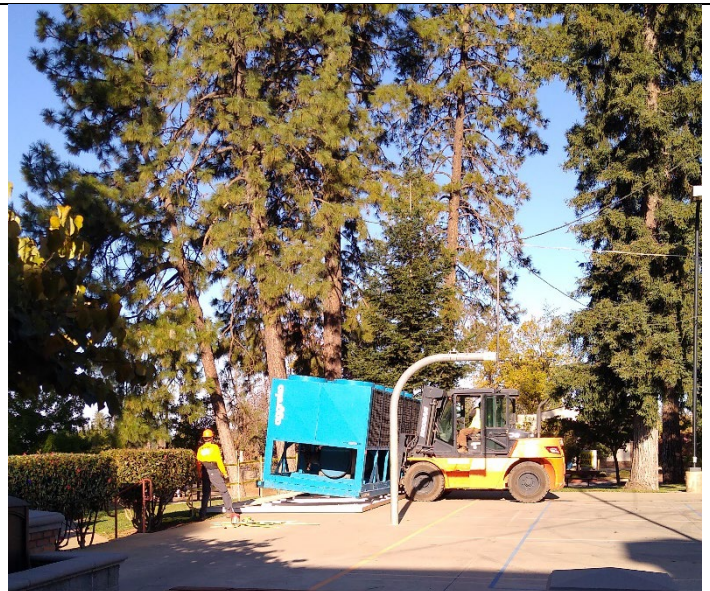
Figure 4. Parks Foreman Lockridge setting the chiller into place.
