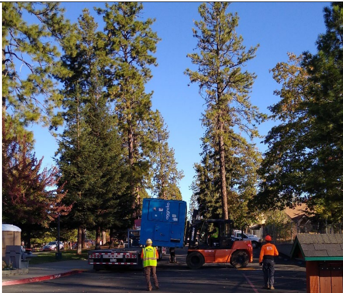
Figure 3. Unloading the chiller.
