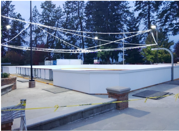
Figure 5. Ice Rink after setup and lighting hung.
