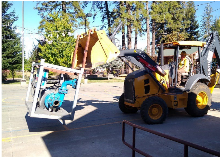
Figure 7. Park Supervisor Cobb driving the chiller motor.
