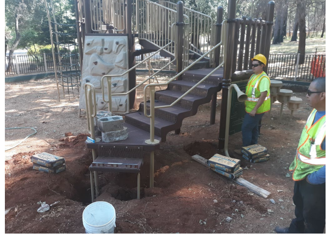
Bille Park Fire Recovery Repairs
