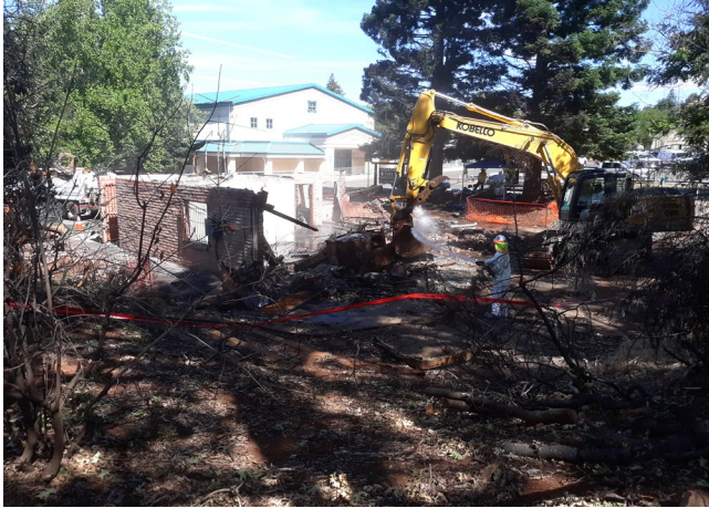
FEMA Pool Recreation Building Demo, July 1, 2019
