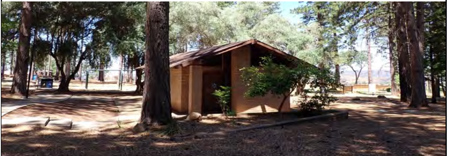
Image 11. Public restrooms in the south.
