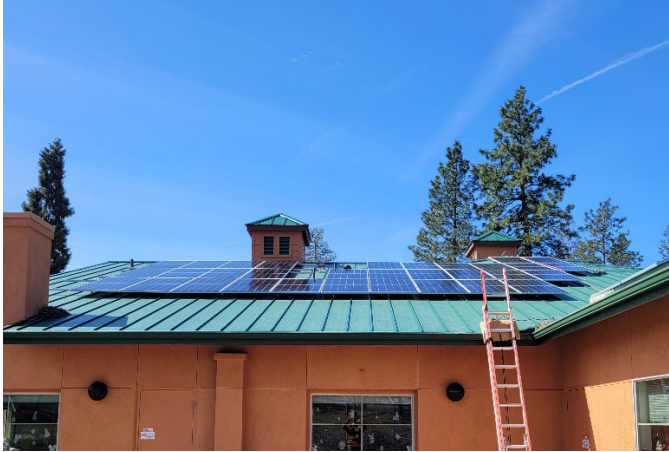
Figure 1. Solar at the TARC is being put up.
