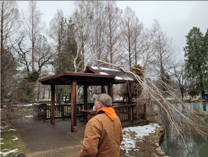
Figure 7. Park Supervisor Cobb assessing more damage at the Aquatic Park.
